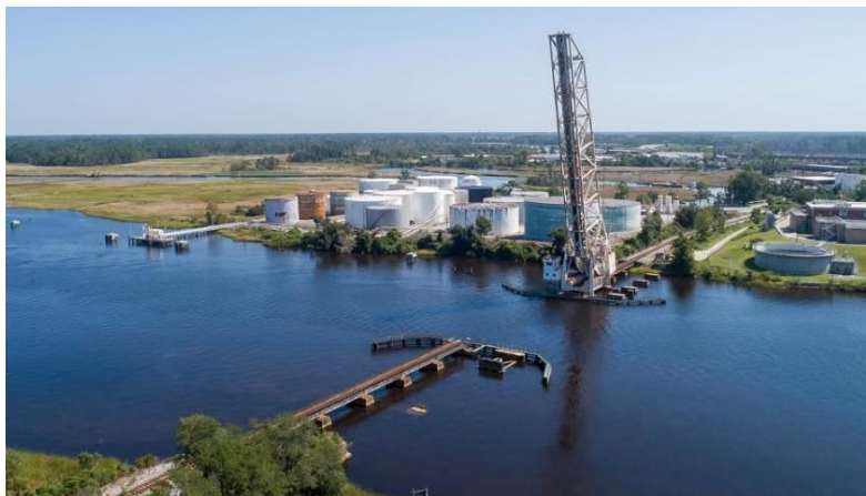
Hilton RR Bridge, Wilmington, a part of the STRACNET Corridor Photo (c) Wilmington Star-News
