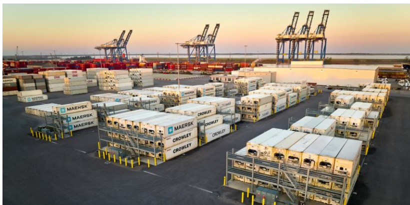
Refrigerated Containers in purpose-built, powered stacks at the Port of Wilmington. Photo (c) NC Ports
